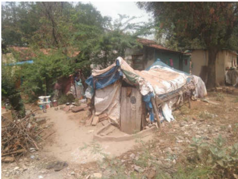
Damaged houses -owners reside in nearby villages
